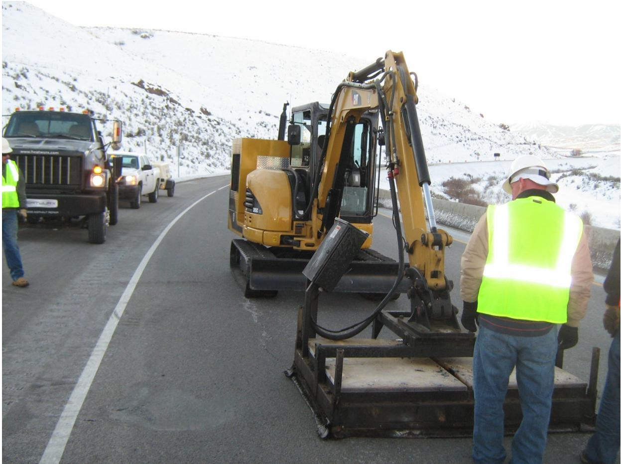
**Figure 3. HeatWurx<sup>®</sup> Infrared Pavement Patching System** Bridge deck pothole repair on I-84 near Echo Junction, Utah. Temperature -5° F.
