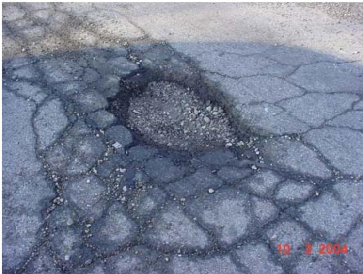
**Figure 1.** Typical pothole showing saturated area around unsealed cracks
