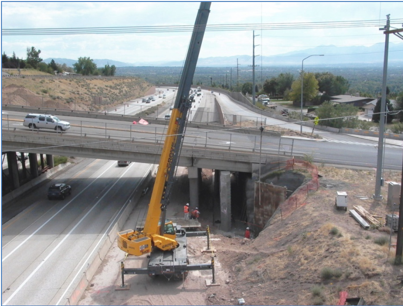
Figure 2 Construction of New Abutments Underneath Existing Structure
