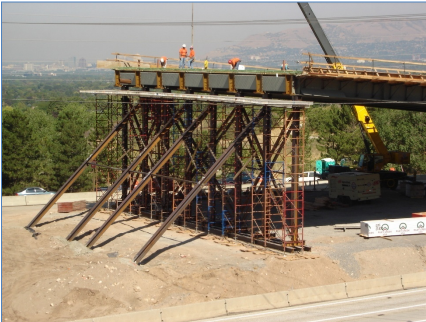
Figure 3 Temporary Abutments
