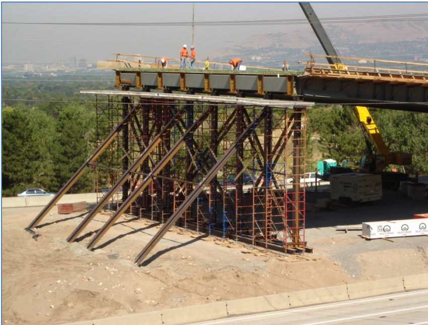
Figure 3 Temporary Abutments
