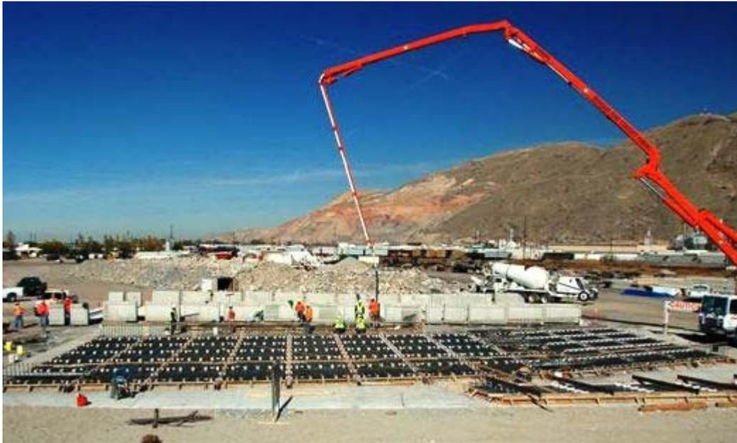
**Figure 3 Precast Yard - Expedites the Installation Process**
