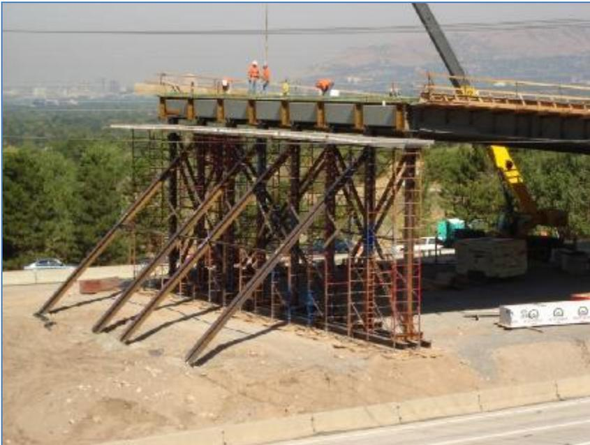
Figure 3 Temporary Abutments
