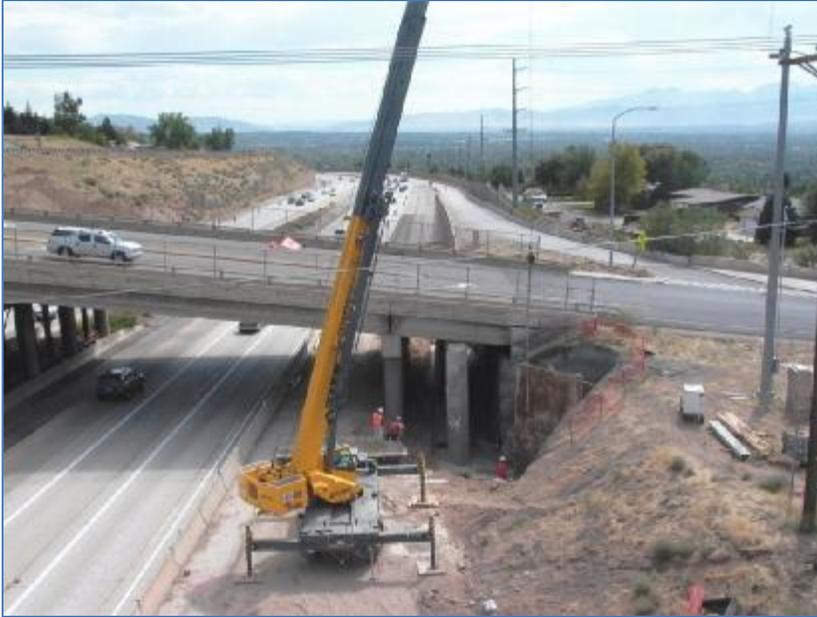
Figure 2 Construction of New Abutments Underneath Existing Structure
