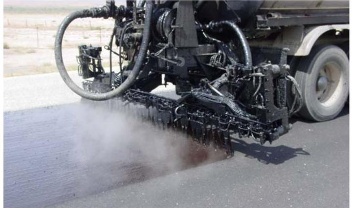
Asphalt is made up of about 95% aggregate (sand, gravel, crushed stone) and 5% binder. The binder is made of asphalt cement and is used to bind the aggregate together. It is used to form a strong, durable surface for roads and highways. In chip-seal applications, the binder must be applied in a specific sequence.
