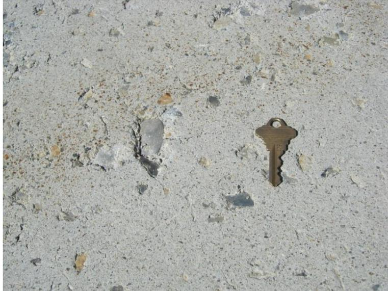
**Figure 2-1 Salt scaling.**
