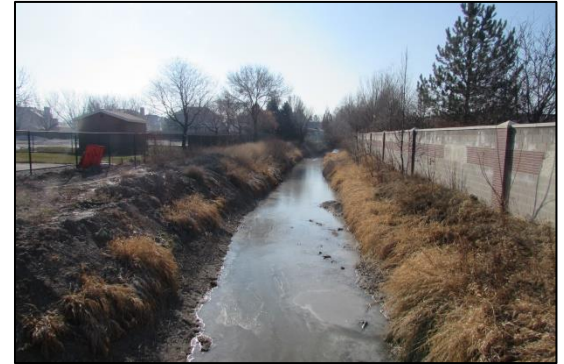
42SL290; East Jordan Canal at 11400 South; view to the south
