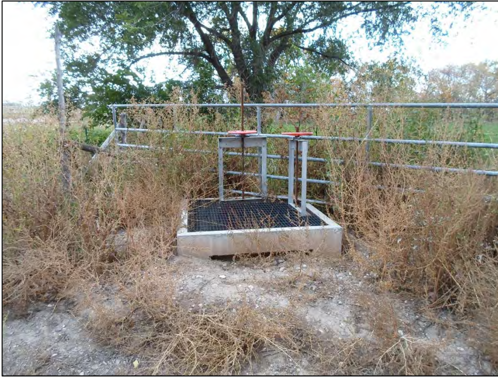
Photo 37. Headgate at the south end of ditch D10 that controls the flow.
